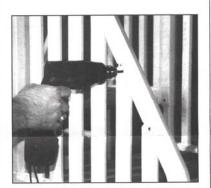
Align one of the triple pickets into the notches of the handrail at the top of the unit. Fasten the pickets in place, at the top of the pickets, using the #10  $\times$  3/4" screws. Continue placing and fastening the double pickets and then the single picket. Repeat for the opposite handrail. Cover the ends of the screws with the protective caps.
